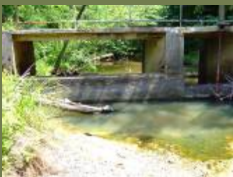
Dam Site at Rice Center
