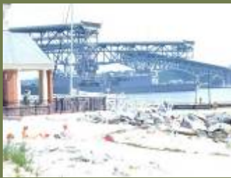
Yorktown Shoreline Protection Project Post Hurricane Isabel
