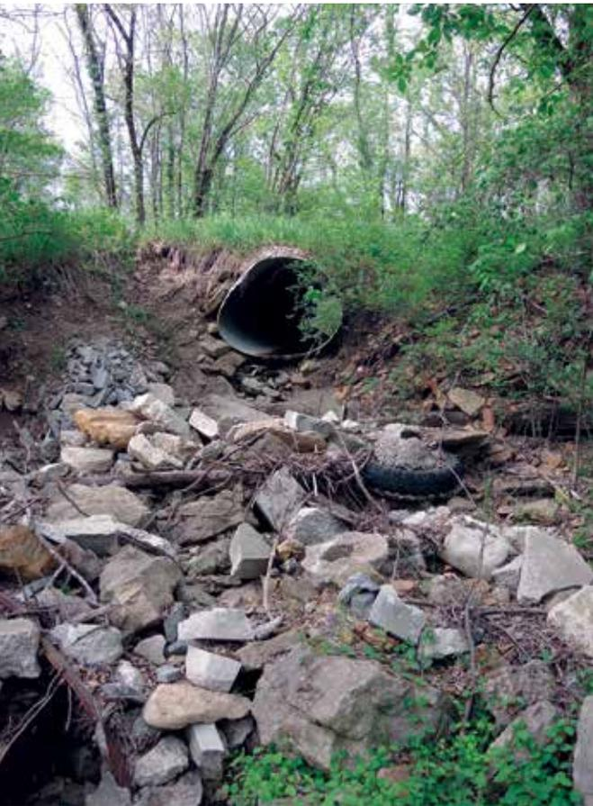
*Figure 2: Many culverts across the U.S. are poorly maintained and are undersized to manage increasing precipitation volumes, resulting in downcutting and erosion. Photo credit: Jeanne Christie, ASWM.*
