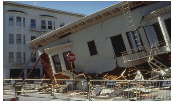
Figure 2. Many floodplains are subject to multiple hazards such as unstable soils and liquefaction which caused building collapse here in the Marina District of San Francisco in the Loma Pietra earthquake of 1989. From https://www.geology.ucdavis.edu/iy (U Davis Geology website).
