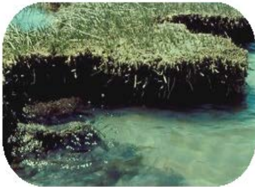
Erosion due to storm waves
