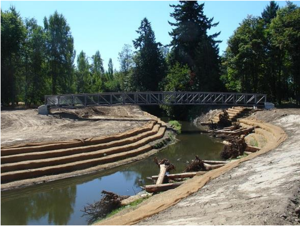
Johnson Creek Pedestrian Bridge
