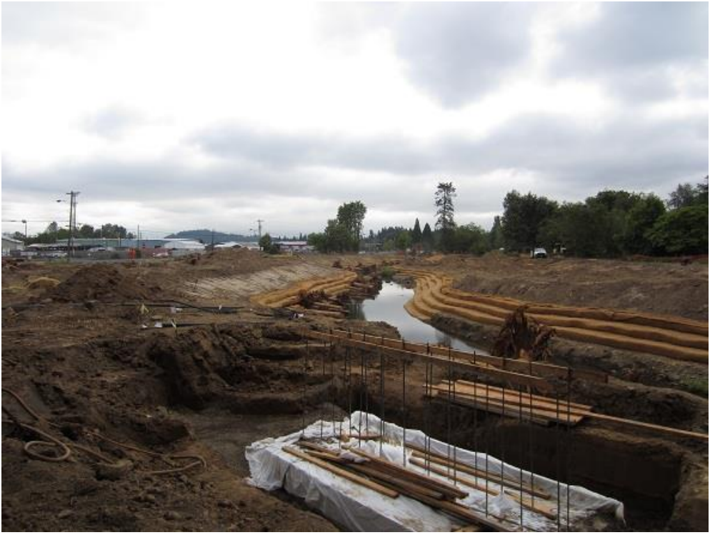
Restored Johnson Creek Bank in East Lents
